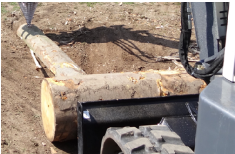
Logs in front of the excavator guard to protect against impact
